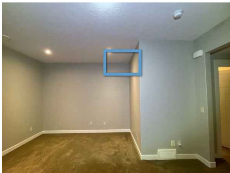
Basement Right Side
