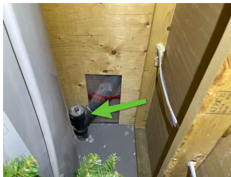
Plumbing Clean-Out: Location Basement, Mechanical Room
