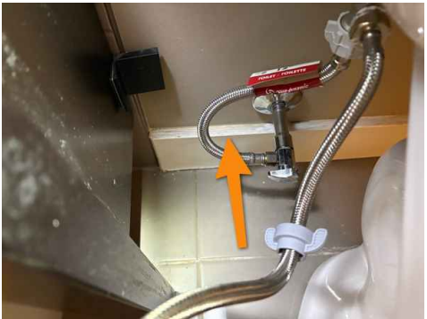
2nd Floor Bathroom
