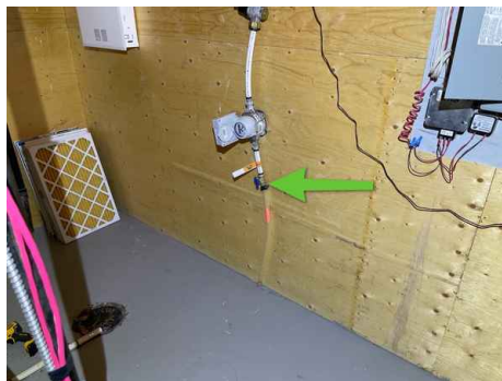
Plumbing Clean-Out: Location Basement, Mechanical Room
