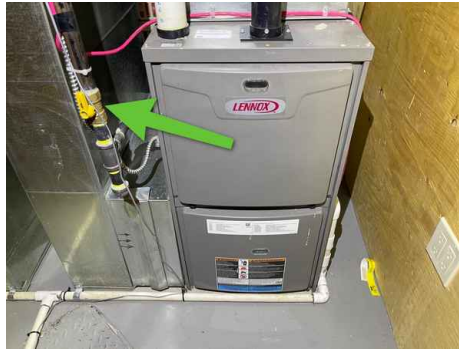
Heating System 2: Humidifier Water Shutoff Above Water Heater
