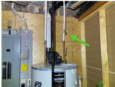
Main Water Shutoff: Location Basement, Mechanical Room
