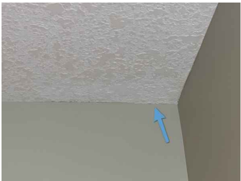
Basement Right Side
